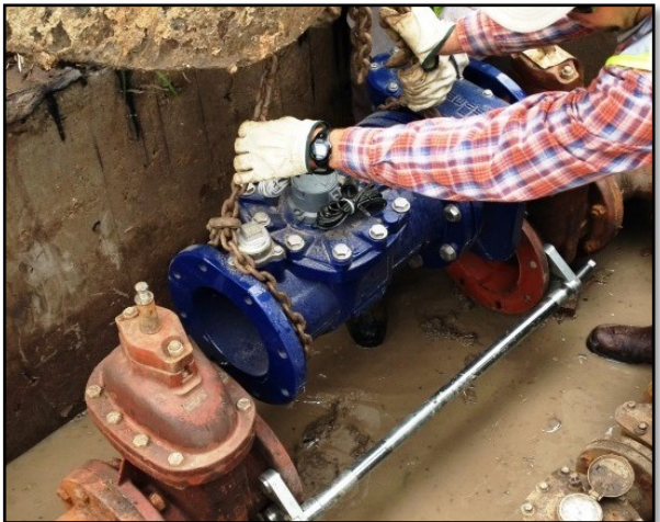
New Meter Installed
